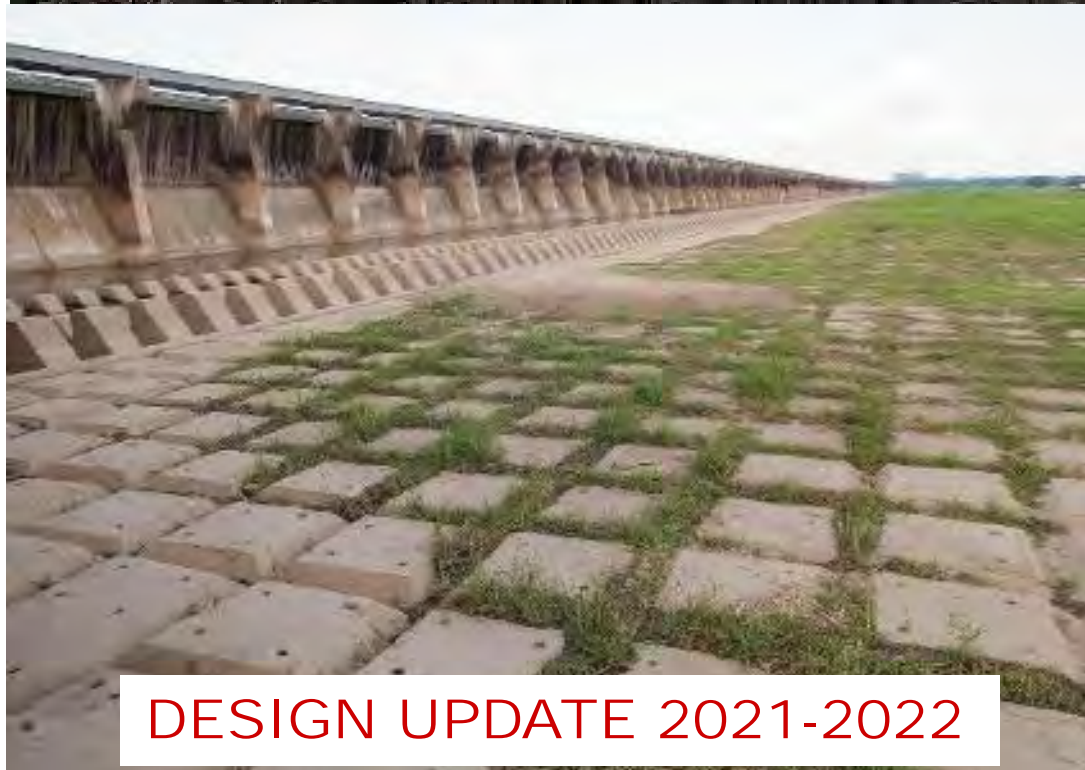
Articulated Concrete Block Mattress Channel Bottom
