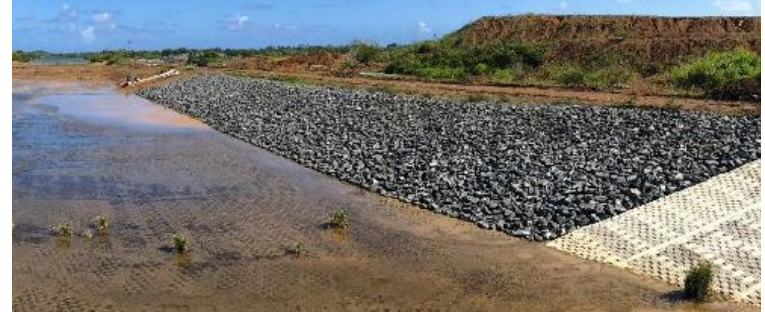
Río de la Plata Channel Bank Stabilization
